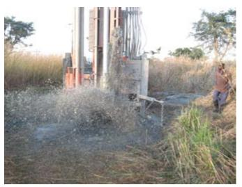
Water sprays as the mammoth drill hits 40 meters depth ... and the beginning of a new well has begun.
